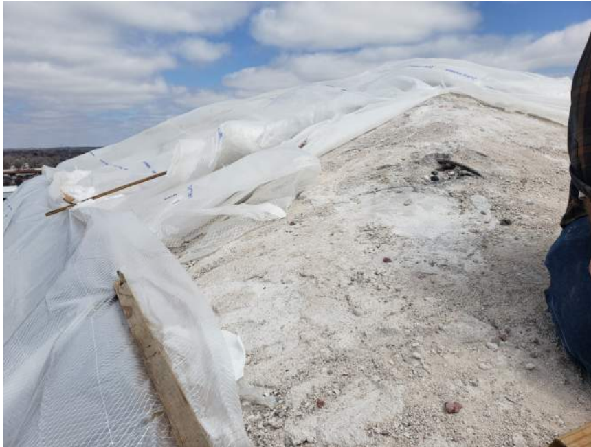
Figure 15. Southwest quadrant of the dome cap exposed.
